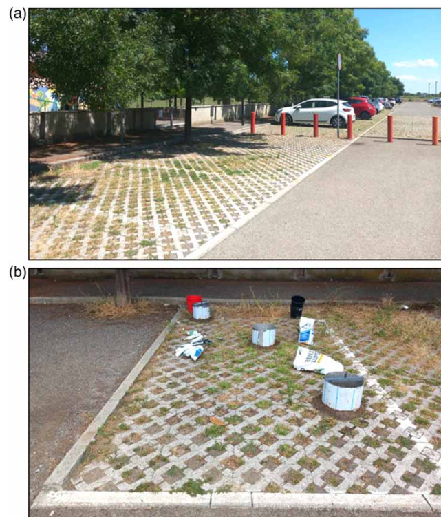
Figure 4 | CGP parking area (a) and experimental set-up (b).
