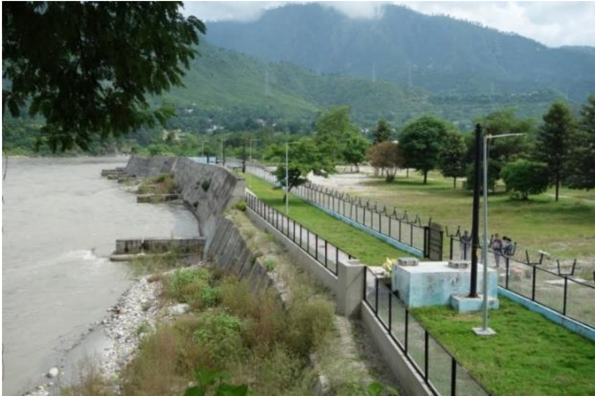
First flood-proof river bank filtration well in Srinagar, Uttarakhand, India. After a severe flood in 2013, a concept to construct flood-proof wells has been developed (NIRWINDU project) and realized in 2017 to protect city drinking water supplies. ( Photo courtesy of F. Musche, HTWD )
