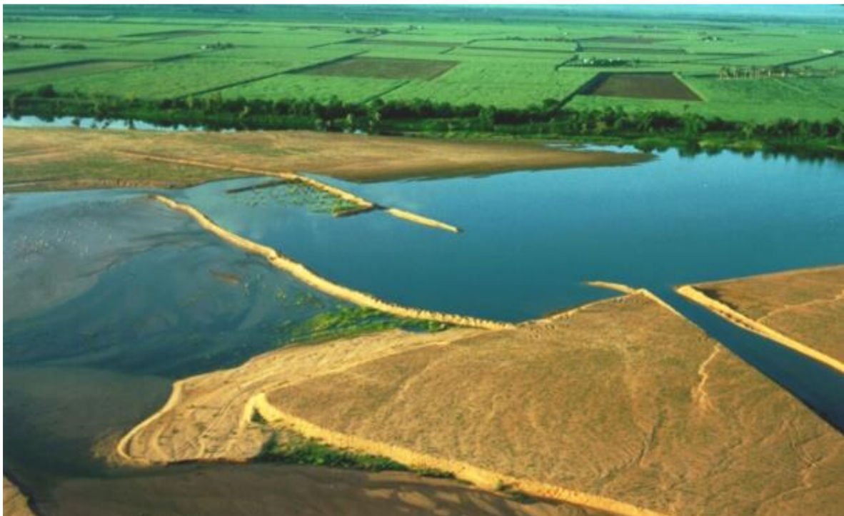
Sand dams in the Burdekin River, Queensland, Australia, to spread water and increase recharge to aquifers used for irrigation supplies. Recharge channels and pits are also used in this area. About 40 Mm 3 has been recharged annually since the 1970s. ( Photo courtesy of Keith Bristow, CSIRO ).
